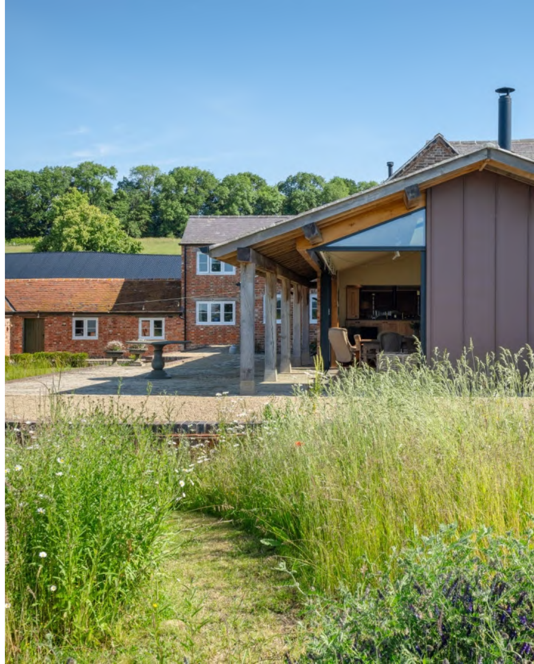
Farmhouse, remodel and addition, Northamptonshire
